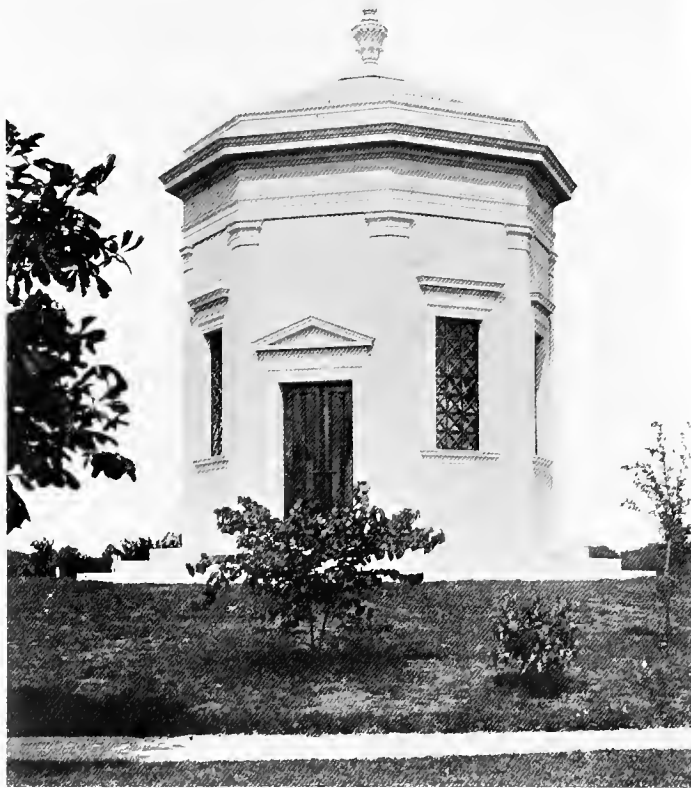
Number 8991. This Memorial Chapel of octagonal form was erected in Woodlawn Cemetery, N. Y., for Mr. Robert Graves. To further insure its permanency, the usual marble lining was omitted and an interior finish given directly to the granite walls. A marble sarcophagus of heavy construction contains two interment receptacles. Memoriae or Mortuary Chapels containing one or more sarcophagi were frequently erected by the Early Christians.
